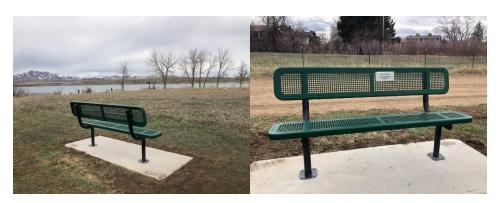
Benches will be 6' long park bench and are made of expanded metal PVC coated. Please allow12 weeks for bench delivery. The bench pad is 4'6" deep x 8' long x 4' thick concrete and padmust cure 2-4 weeks before bench can be installed.
